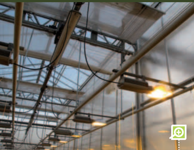
Figure 10: High pressure sodium lamps in a greenhouse
